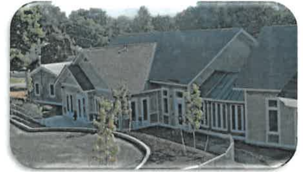
West Street Center ~ North Bennington
