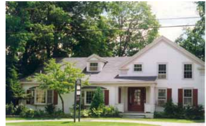
The Stephen C. Lundy Building, Manchester
